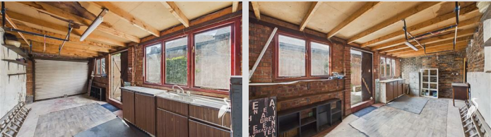
Base units incorporating a single bowl stainless steel sink and drainer. Accessed via roller shutter door. Single glazed windows and door to rear garden.
